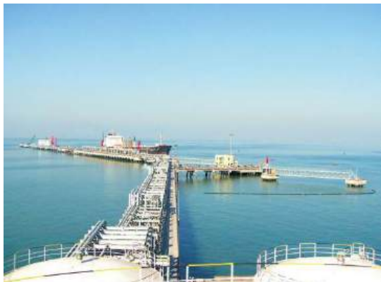
Ham Petrol Boru Hattı - Crude oil pipeline
