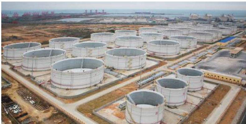
Ham petrol depolama tesisleri - Crude oil tank farm
